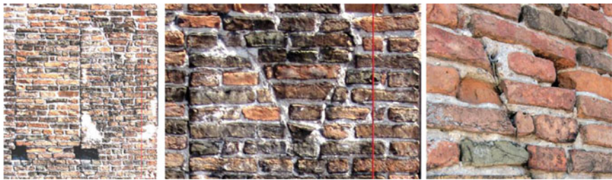
Fig. 5 Probable merlons embedded in the masonry texture
