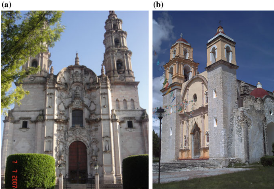
Fig. 1 Typical colonial churches built in: a low seismic risk zone (central Mexico), b high seismic risk zone (Pacific coast)
