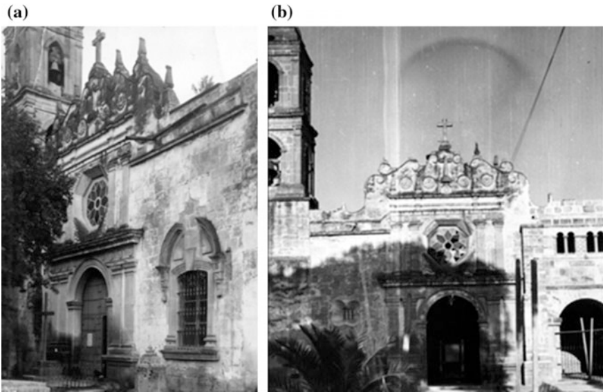
Fig. 8 View of the Façade in the of the past century [11], decade of: a 40s; b 50s
