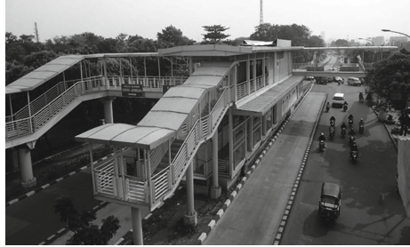
Fig. 2. A typical design and location of the TransJakarta BRT station
