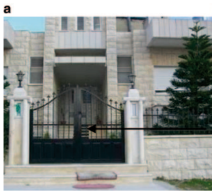
a Stairs are constructed on the sidewalk in front of the gate.
