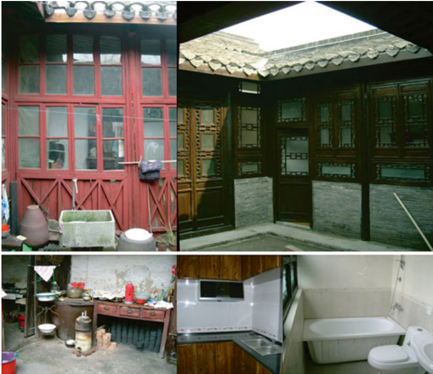
Fig. 19.8 Pilot project house in Yangzhou before ( left ) and after renovation ( right ) (Source: GTZ Project Team)
