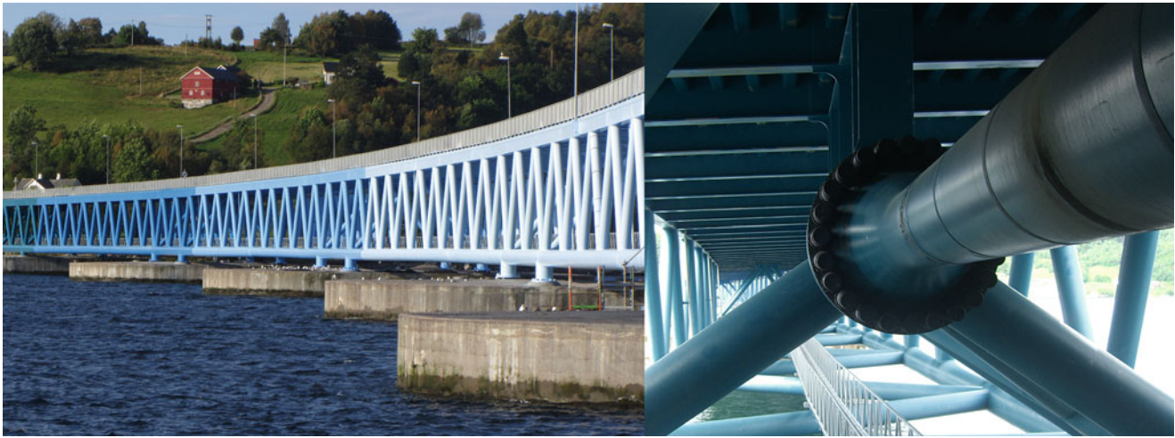
Fig. 14.1 Left: the Bergsøysund Bridge. Right: one of the two steel rods taking all axial action at the abutments
