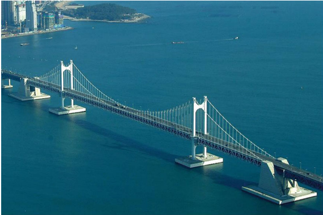
Fig. 11.1 An overview of the Gwang-An bridge
