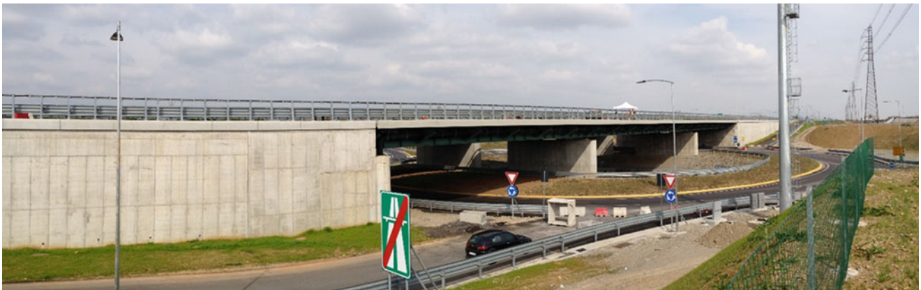
Fig. 17.1 VX bridge: view
