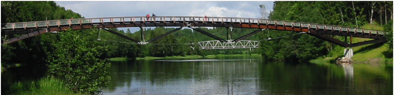
Fig. 9.1 The Lardal Bridge, built in 2001, with a total length of 130 m as it crosses the river Lågen in Norway
