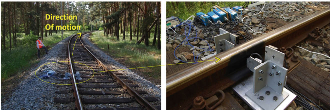
Fig. 20.9 Portable measurement device placement during 600 m radius curve tests
