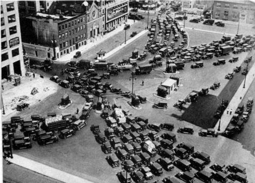
Fig. 4.1 Holland Tunnel Bottleneck (1940)—27 lanes trying to get into 2 lanes. Source Reference [4], p 110
