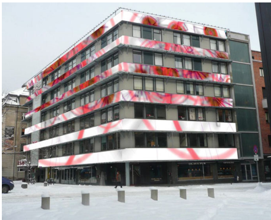
Facade Norway . 2010. Live data visualisation connecting the city using sensors
