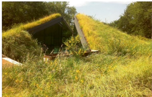
Fig. 3.9 Green roof on a residential building in Texas (Green Roof: Ecosystem Design Group, Lady Bird Johnson Wildflower Center, University of Texas at Austin Architects: Bercy Chen Studio LP)
