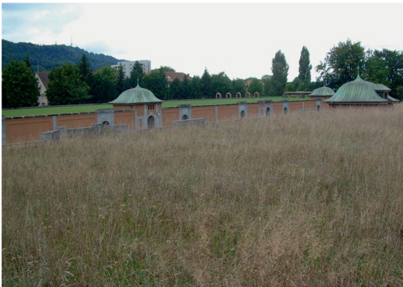
Fig. 13.4 The Moos Lake water filtration plant in Willishofen, Zürich, Switzerland was built in 1914 and is home to 175 plant species, many of which are now endangered or rare. (Photo DB Rowe)
