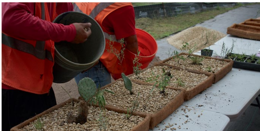
Fig. 16.11 Biodegradable coconut fiber trays were filled with a substrate mix of 20% natural soil (from nearby Fort Worth Prairie) and 80% engineered substrate in the trays and then 100% engineered substrate below the trays. Trays (above) are being planted with pre-grown plants in plug form including the Opuntia phaeacantha (Prickly Pear cactus) indigenous to the Grand Prairie. (Botanical Research Institute of Texas)
