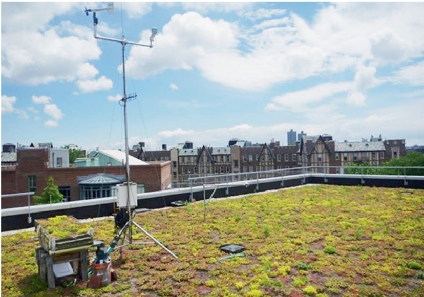
Fig. 2.10 Meteorological and hydrological monitoring at the Ethical Culture Fieldston School green roof (Kimberly DiGiovanni)
