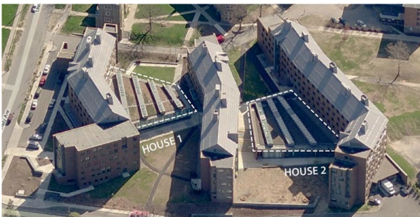
Fig. 12.3 The green roofs examined in this case study are the Alice H. Cook House (House 1, left), an intensive roof, and the Carl L. Becker House (House 2, right), an extensive roof. (Bing Maps, Image modified by KieranTimberlake)
