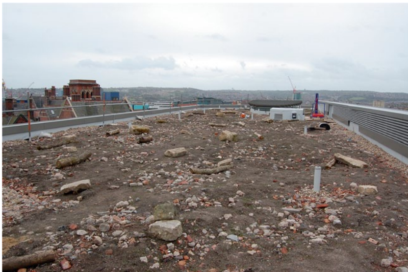
Fig. 10.2 Mixed growing substrate, a variety of textures and aggregate sizes, and varying growing media depths, spread over a green roof prior to encouraging colonization by ruderal species. ( Nigel Dunnnett )
