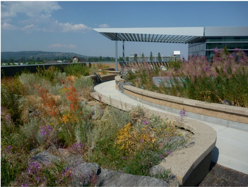
Fig. 4.4 The green roof on top of the Oregon Dental Service (ODS) Building in Bend, OR. In extreme water environments like Bend, designs may need to incorporate deeper substrate depths if diverse vegetation is a goal. Substrate depths here vary from 20 to 81 cm (8–32 in.). (Photo: Richard Martinson)
