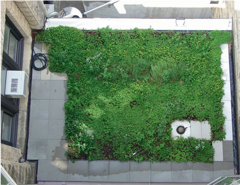
Fig. 16.2 Lower Seaton Hall Green Roof at Kansas State University assembled from LiveRoof™ modules. The modules are populated with 11 species of prairie plants installed in 2012 and some replanting in 2014. (Lee R. Skabelund)
