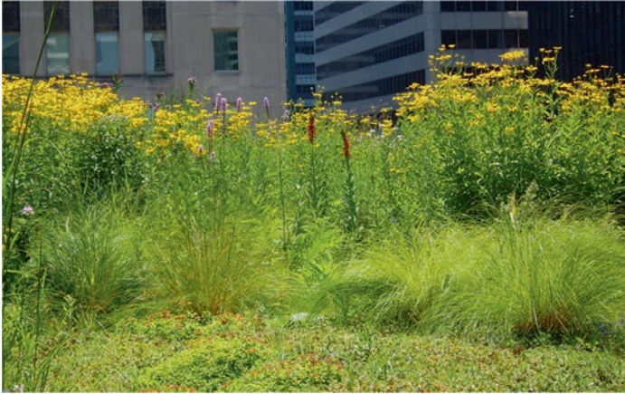
Fig. 16.20 Initially planted with bands of plants extending across semi-intensive (background) and extensive (foreground) substrates, plant species have now sorted to their preferred microclimates on the roof. (Bruce Dvorak)
