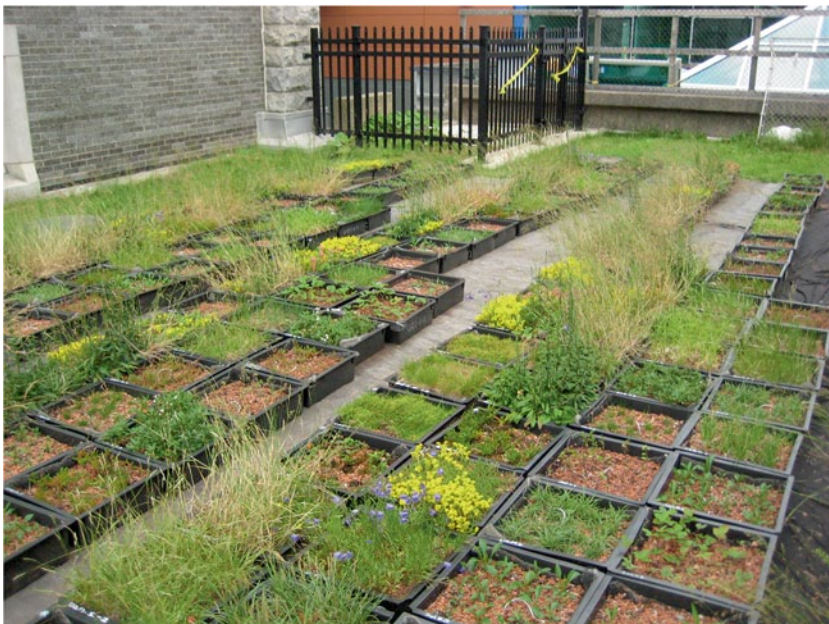
Fig. 16.14 The modular green roof plots where plant, temperature, evaporation and plant combination research has taken place on the St. Mary’s University in Halifax. (Jeremy Lundholm)
