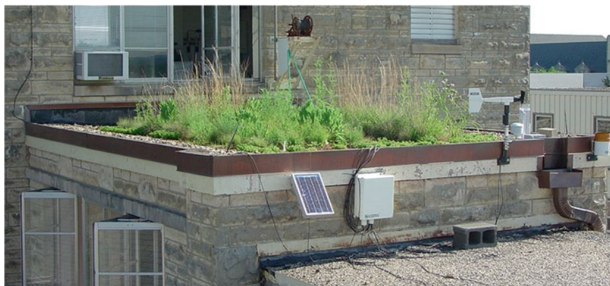
Fig. 16.3 Monitoring equipment set up on the Upper Seaton Hall Green Roof in June 2009 to capture temperature profiles, stormwater runoff, precipitation, wind speed and direction, relative humidity, and air temperature. (Lee R. Skabelund)
