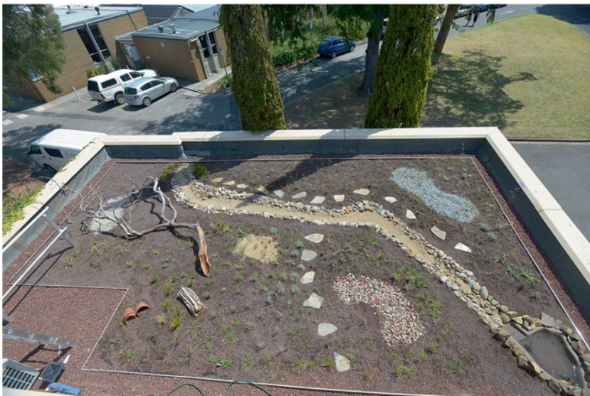
Fig. 16.5 Bio-diversity roof includes a small pond, water channel, wood and rock debris to attract local fauna. (Les O'Rourke)
