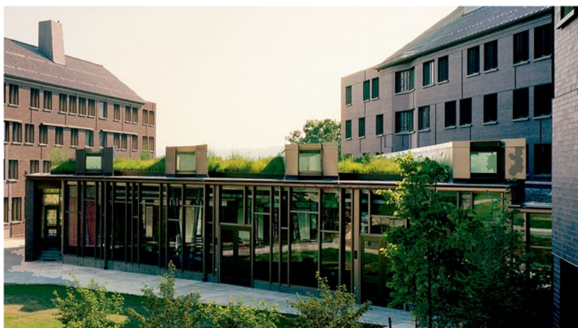
Fig. 16.12 Meadow and early pioneer vegetation established on the Alice H. Cook House at Cornell University. The green roof is left to natural succession, as it has not had any human interference regarding removing of species or active maintenance, with the exception of irrigation during the first year of plant establishment. These conditions have allowed for observation of species interactions, dynamics and dominance on the roof. (Halkin Mason Photography)
