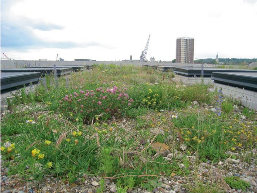
Fig. 16.17 Bio-diverse roofs give rise to a range of pioneering meadow plants, mosses, lichens, and other life-forms adapted to disturbed urban conditions without irrigation or maintenance. This photo of the Laban Center roof was taken eight years after completion, and is good habitat for arthropods such as spiders. (Dusty Gedge)
