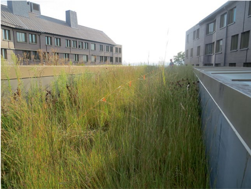
Fig. 16.13 Detailed plant surveys of the green roofs relied on dozens of Relevé (concise summaries of distinct vegetative units) over 7 years. Vegetation on the Alice H. Cook House during 2012, a growing season with drought conditions. (Stephanie Carlisle)
