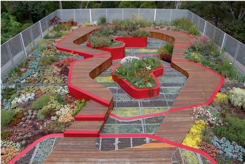
Fig. 16.4 Burnley demonstration green roof demonstrates fourteen (14) different planting zones, each with different microclimates and habitats made from ascending substrate depths (front to back), watering treatments, moisture gradients and plant communities. (Les O'Rourke)
