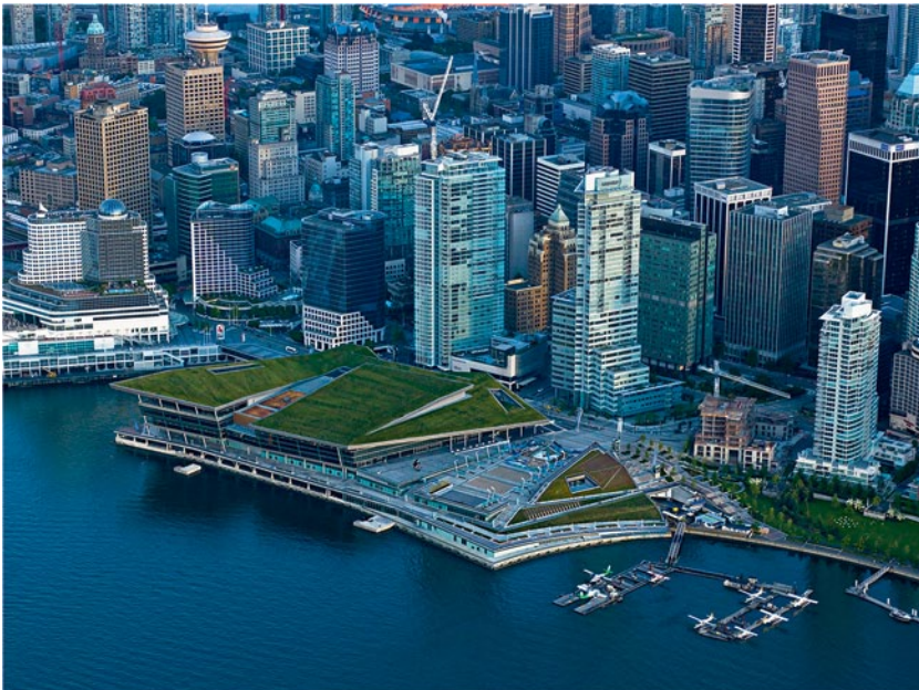
Fig. 16.6 Green roof coastal meadow ecosystem covers the sloped rooftops of the Vancouver Convention Center. The nearly 2.5 ha installation over multiple levels of green roofs and public decks manifest an elegant and seamless integration of ground level vegetation rising to the rooftops. The Vancouver skyline is in the background and overlooks the green roof meadows, Waterfront Park and Vancouver Harbor. (PWL Partnership Landscape Architects Inc.)
