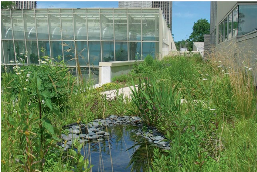
Fig. 16.1 Wetland, mesic and upland prairie green roof at the Peggy Notebaert Nature Museum in Chicago, Illinois. Over 100 native plant genera were installed in 2001. Substrate depth increases from 15 cm for the wetland ( foreground ) to 45 cm for the prairie ( background ). (Conservation Design Forum Elmhurst, IL)
