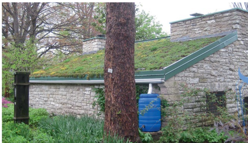
Fig. 16.9 Stormwater runoff from the Cottage House Green Roof (shown here) is sampled for flow rate and chemical analysis of runoff. (Ishi Buffam)
