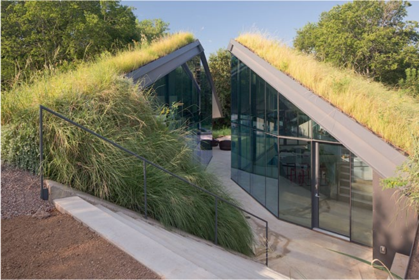
Fig. 16.18 Blackland Prairie plant species extend from the ground up to the vegetated and sloped rooftop for a seamless integration of land, structure and prairie. (Copyright Paul Bardagjy)
