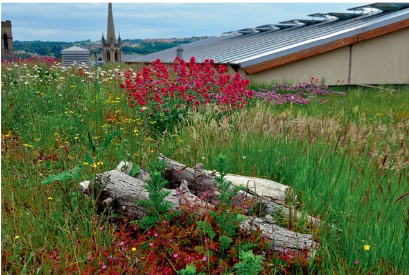
Fig. 10.1 Green roof vegetation created through spontaneous colonization, with log pile (Nigel Dunnett) (Sharrow School Green roof, Sheffield)
