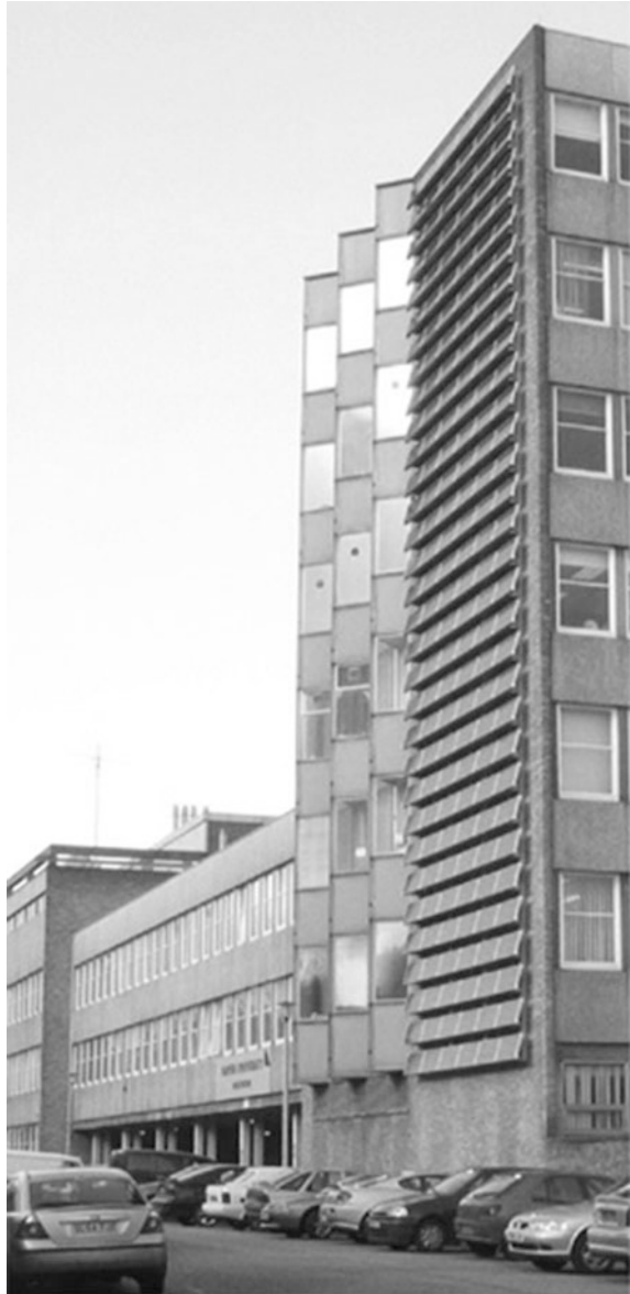
Fig. 8 Solar panels installed on the southeast face of the Edinburgh Napier University —Merchiston campus
