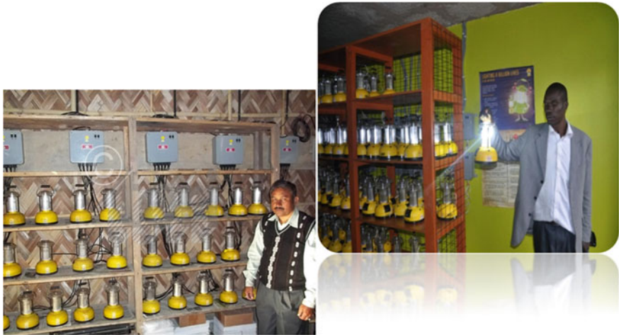
Fig. 6 A solar charging station implemented in India and Africa. Source: TERI
