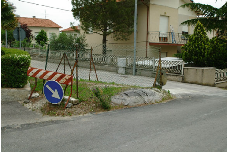
Fig. 6.2 A temporary repair undertaken due to rising gas and mud after the plumbing of the ground at a cross road in Serra dé Conti village (central Italy) ( photo by L. Innocenzi, INGV)
