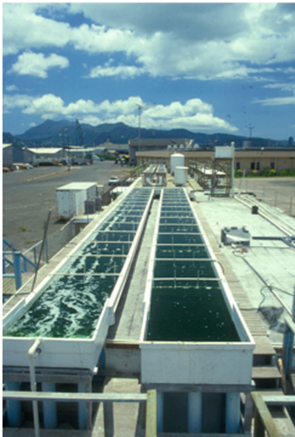
Fig. 30 Microalgal culture facility at the UH Marine Center (Photo: Dr. Edward Laws, LSU School of the Coast and Environment)
