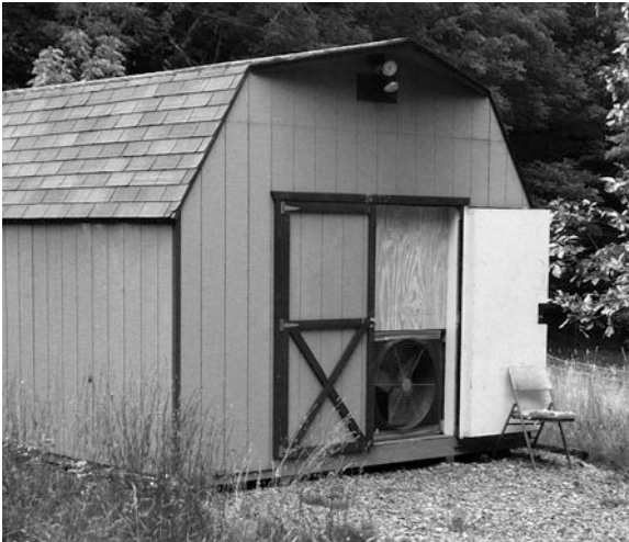
Fig. 22.14 Inside this shed used for apple storage is Big Bucks Pit, a 43 m drop into Barberry Cave. The pit is sealed to the floor of the building. The door to the building has been reduced to the size of the fan. Accordingly, as the fan blows in and out of the building the air is exchanged in the cave (photo by P. C. Lucas)
