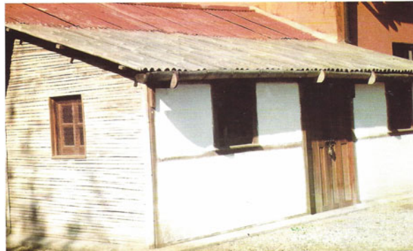
Fig. 9.17 Plastering of bamboo mat walls, India (Liese and Kumar 2003)
