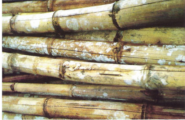
Fig. 9.1 Cracks during storage with subsequent fungal decay (Liese and Kumar 2003)
