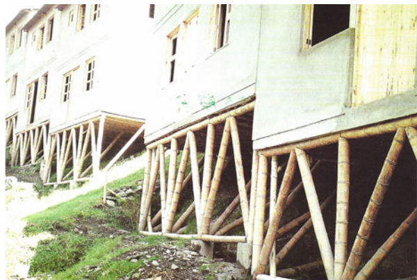
Fig. 9.21 Social housing programme with bamboo houses in Manizales, Colombia (Liese and Kumar 2003)
