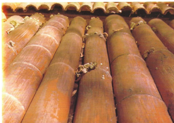
Fig. 9.22 Fruit bodies indicate advanced decay of a bamboo roof (Liese and Kumar 2003)
