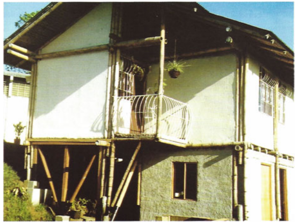
Fig. 9.19 Bamboo house with plastered walls in Costa Rica (Liese and Kumar 2003)
