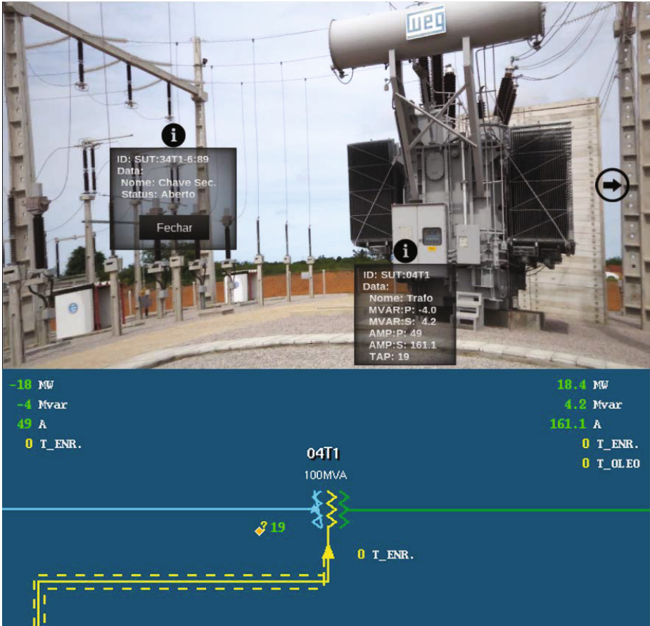
Fig. 5. Panorama of a substation visualized in PS-PAE showing real time information retrieved from SAGE
