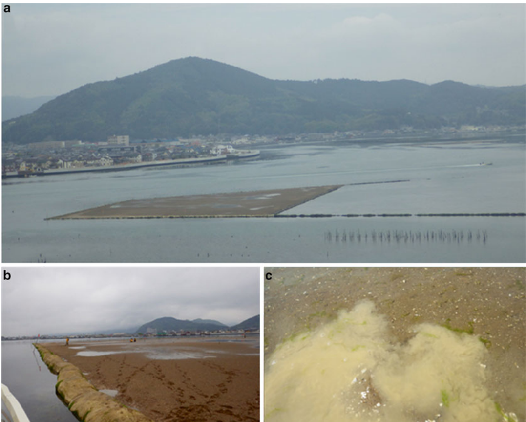
Fig. 6 (a and b) Artificial tidal flats made by mountain sediment in Mangoku-ura Inlet; (c) Turbidity occurs when stir the newly-introduced mountain sediment
