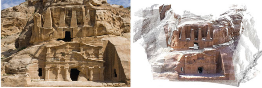
Fig. 12.22 View of the obelisk tomb and the Bab As-Siq triclinium in Petra/Jordan and a 3D view of the four-point clouds collected [29]
