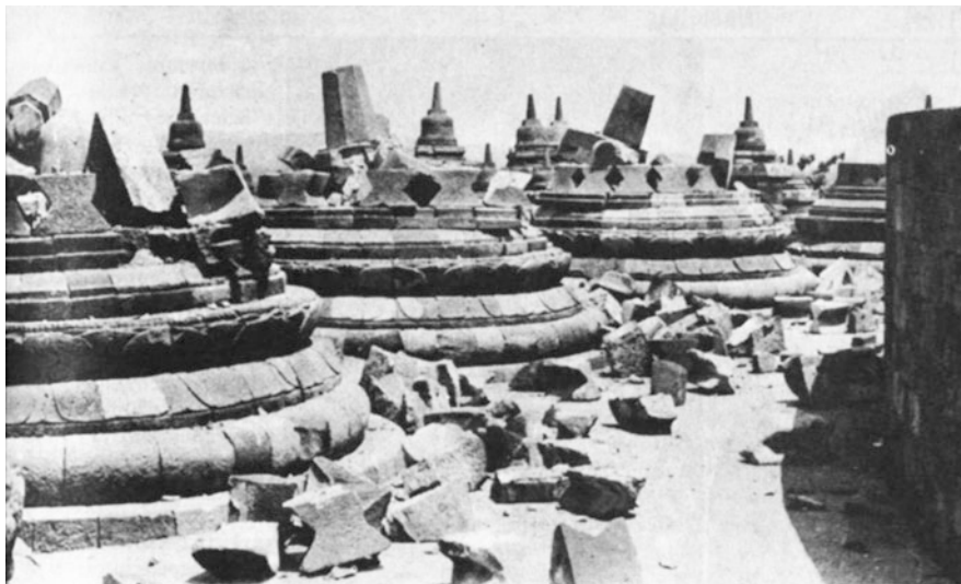
Fig. 5 Damage caused by the bomb attack at Borobudur, January 20/21, 1985 (Source: Ledakan 1985)
