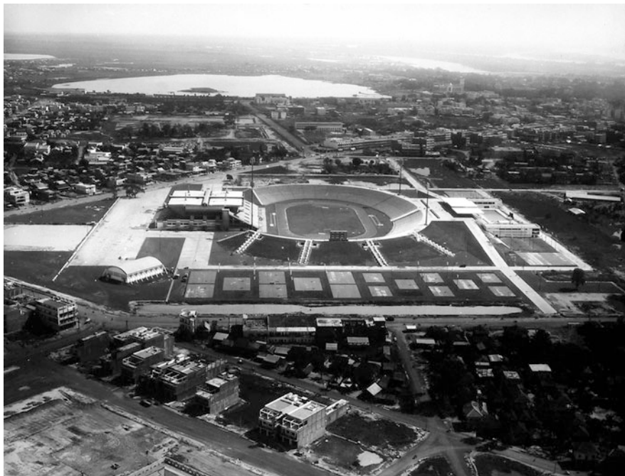
Fig. 14 National Sports Complex, Phnom Penh, inaugurated on December 12, 1964. In this 1960s aerial picture the “Sports Palace” and “Grandstand” can be seen on the left of the stadium with the “Olympic” podium, swimming pool, and diving pools to the right. Architect: Vann Molyvann (Vann Molyvann)
