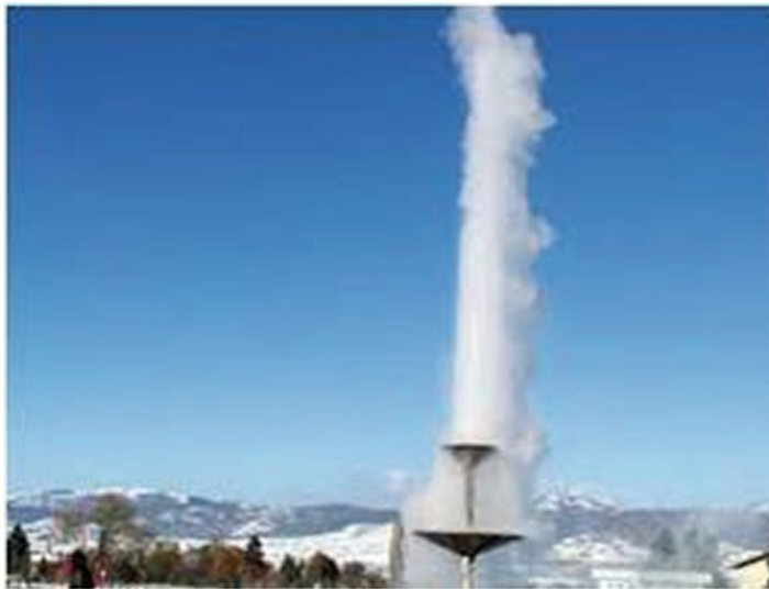
Fig. 4.1 Geysera, Sapareva Banja, Bulgaria is characterized by water temperature of 103 °C in the hole drilling
