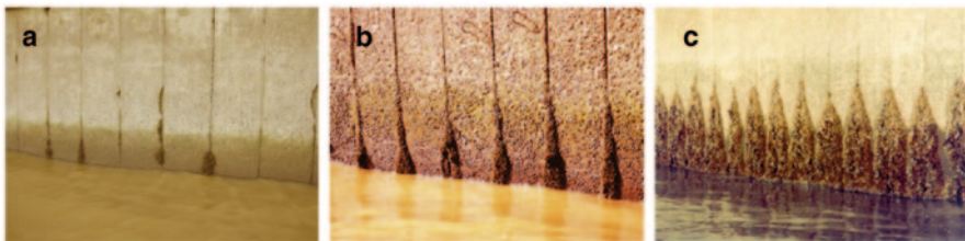
Fig. 4 Different degrees of development of mussel beds on pilings along the coast of the Luján River (lower delta of the Paraná River). (From Boltovskoy et al. 2006)
