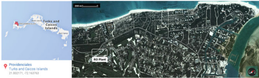
Fig. 9.6 SWRO plant and wells at the Turks & Caicos Water Company, Providenciales, Turks & Caicos Islands (modified from Rachman et al. 2014)
