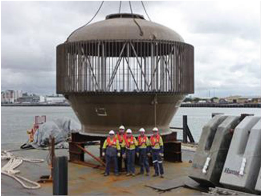
Fig. 3.14 Very large velocity-cap intake structure used at the Gold Coast SWRP plant
