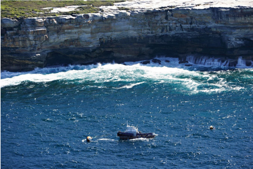
Fig. 2.2 Surge and wave conditions—Sydney desalination plant inlet
