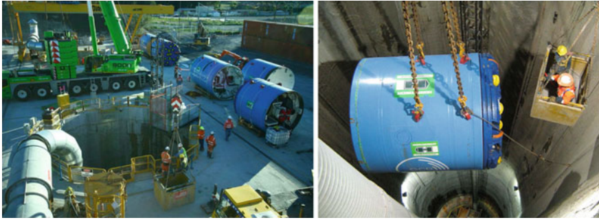
Fig. 2.4 Tunnel access shaft and TBM components/TBM segment being lowered for assembly below ground
