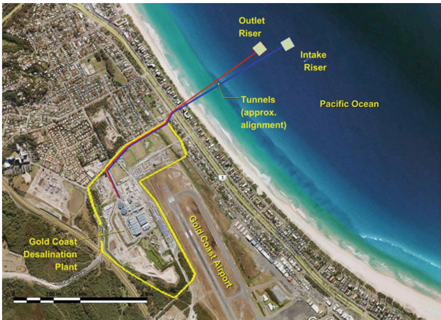
Fig. 2.3 Gold Coast desalination plant—tunnel and marine structures locations
