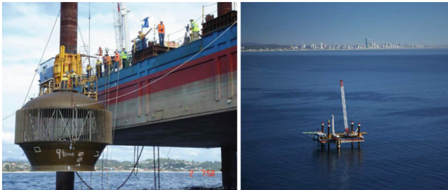
Fig. 2.6 Intake coarse screen being installed from the jack-up barge
