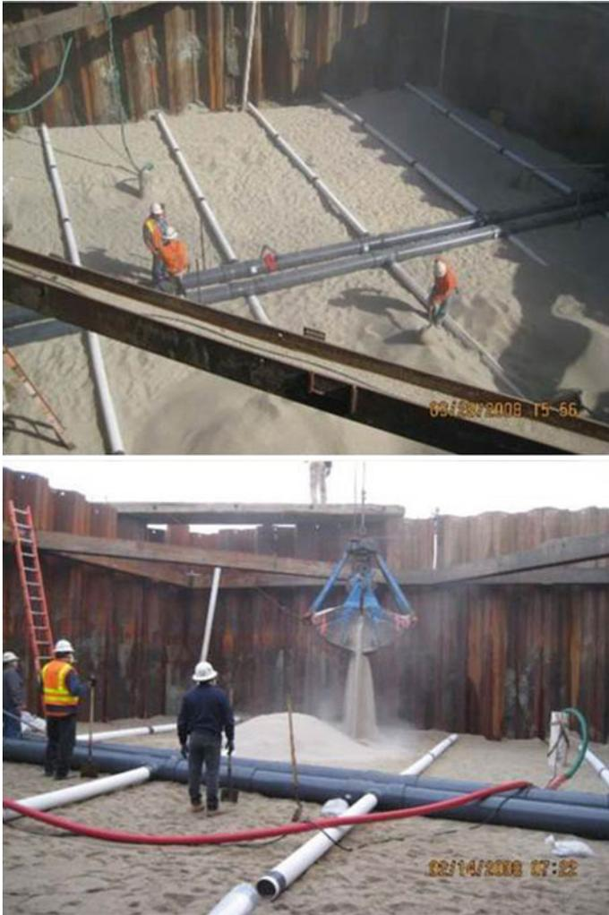
**Fig. 11.14** Construction of the City of Long Beach test seabed gallery cell using sheet piling and dewatering the excavation prior to filter emplacement
