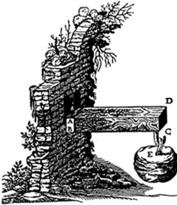
Fig. 3 Galileo's depiction of a beam (1638, p. 114)
