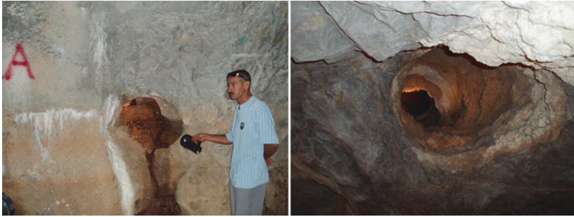
Fig. 3.20 Subhorizontal karstic channel in totally impermeable block of Upper Cretaceous limestones. It functions as a single conductive path for groundwater, but it is able to transfer enormous flow (foundation of the Hammam Grouz dam, Algeria)
