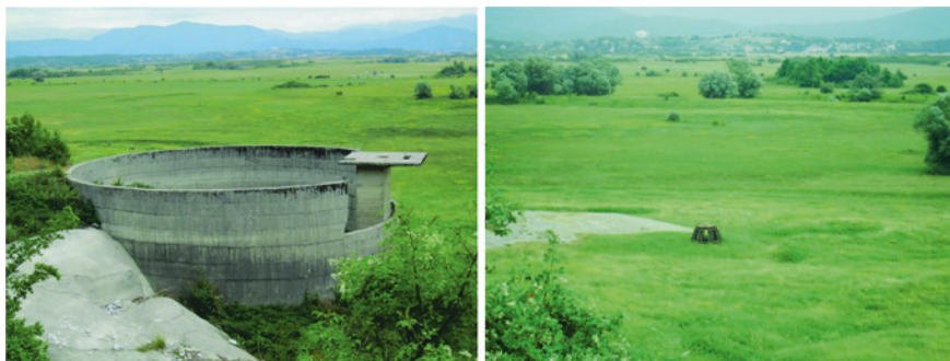
Fig. 16.1 Reinforced concrete cylindrical dam around Opačica ponor (sinkhole) ( left ); non-returned valve constructed on some small sinkhole in the area of Vrtac Reservoir in Nikšić polje ( right )
