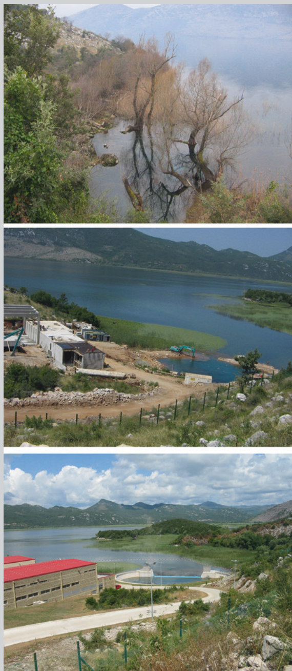
Fig. 16.50 Intake Bolje sestre and three stages of its construction
