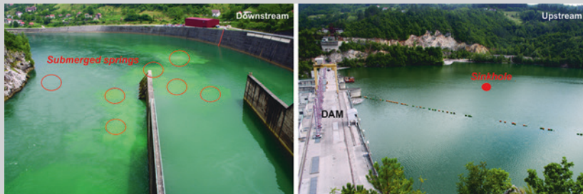
Fig. 16.13 Left —Submerged discharge points during tracer test ( downstream, left photo ); Spatial position of main sinkhole (location of tracer injection at a depth of 50 m) ( upstream/reservoir, right photo )
