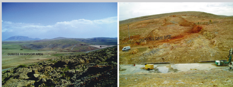
Fig. 16.7 Ourkiss dam site and reservoir area during construction
