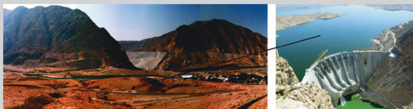
Fig. 16.2 Photo of dam site during construction and Salman Farsi Dam in the last stage of building
