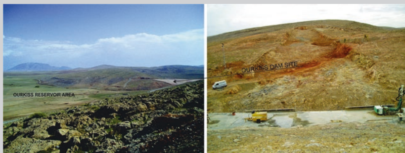
Fig. 16.7 Ourkiss dam site and reservoir area during construction
