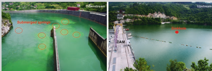
Fig. 16.13 Left —Submerged discharge points during tracer test ( downstream, left photo ); Spatial position of main sinkhole (location of tracer injection at a depth of 50 m) ( upstream/reservoir, right photo )
