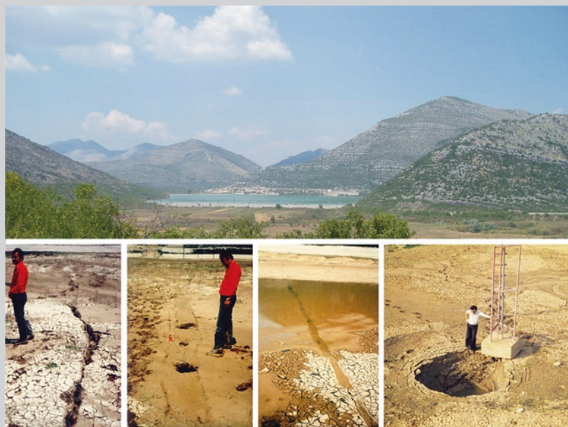
Fig. 13.2 Hutovo reservoir, Herzegovina. Sinkhole and cracks created at the reservoir bottom and beneath protective plastic foil after first reservoir filling. Photos P. Milanović
