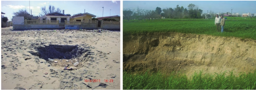
Fig. 17.2 Natural sinkhole (left) and collapse sinkhole (right), the latter being related to presence of an underground quarry
