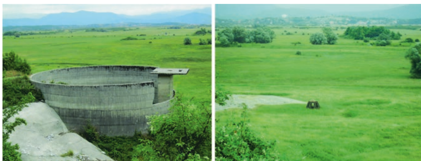
Fig. 16.1 Reinforced concrete cylindrical dam around Opačica ponor (sinkhole) ( left ); non-returned valve constructed on some small sinkhole in the area of Vrtac Reservoir in Nikšić polje ( right )
