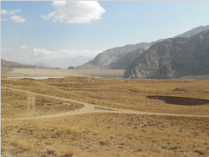
Fig. 13.3 Lar Dam and reservoir, Iran. One of the sinkholes at the reservoir bottom. Photos P. Milanović
