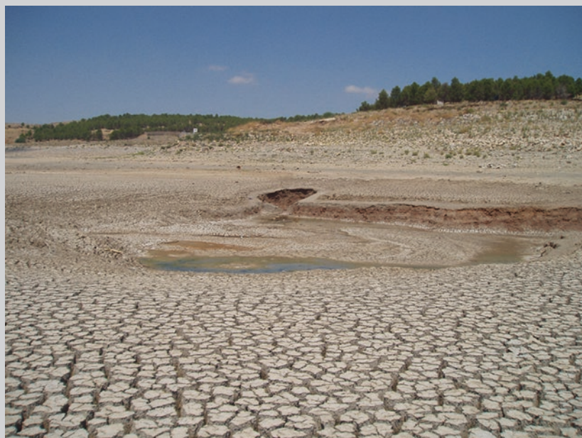
Fig. 13.11 Hammam Grouz reservoir, Algeria. Collaps at reservoir bank occurred after 17 years of operation. Photo P. Milanović
