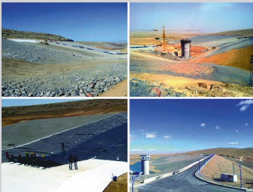
Fig. 16.12 Photos from the phase of impermeable carpet installation (geomembrane and geotextile) http://www.hidrotehnika.rs/alzir/brana-ourkiss/
