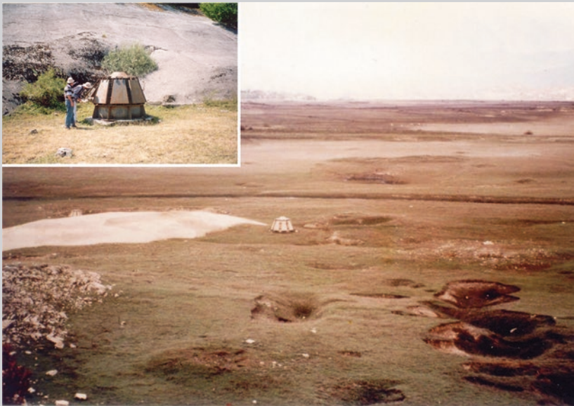
Fig. 13.9 Vrtac reservoir, Montenegro. New estavelles developed during first reservoir filling. Upper left one way valve constructed at estavelle opening. Photos P. Milanović
