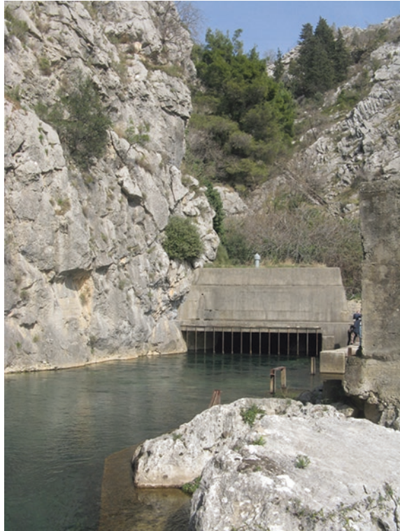
Fig. 11.4 Detail from Jadro Spring (Split, Croatia): concrete barrier placed on main spring orifice (old Roman intake reconstructed in 1885/1886)
