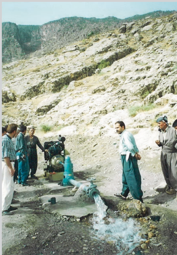
Fig. 6.18 One of the wells drilled in the foothill of karstified limestones (Shaqlawa, north Iraq)
