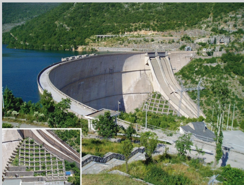
Fig. 13.1 Grančarevo Dam, Herzegovina. Stabilization of left slope by pre-stressed anchors. Photos P. Milanović
