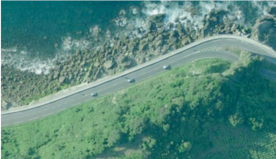
Fig. 1 Overview of Km 22 in N-634 road
