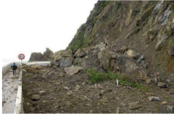
Fig. 2 Landslide occurred in the studied spot on 2008
