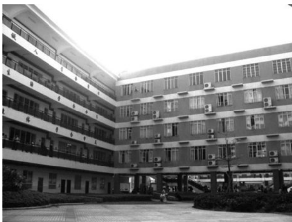
Fig. 13.2 The central courtyard, the teachers' office (where the air conditions are attached), and the classrooms (on the left ) (Photo taken by the author)
