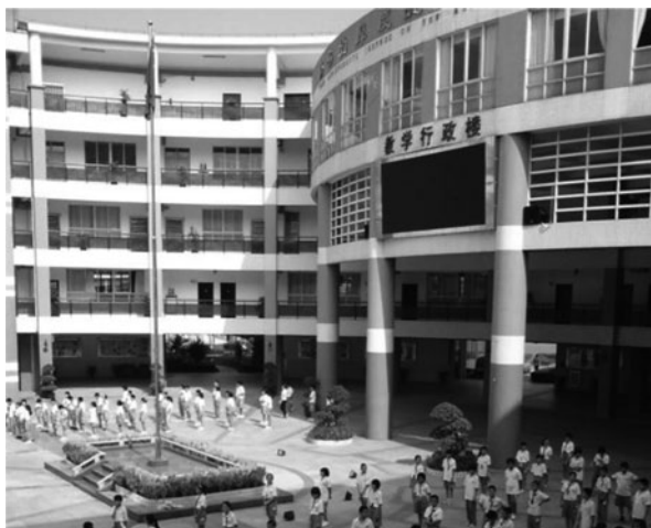
Fig. 13.1 The central playground, the multi-function building, and the administrative offices of the Grand-Estate School (Photo taken by the author)
