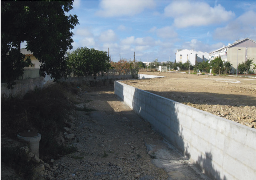
Fig. 6 Concrete walls canalizing the Sassoeiros stream. Such monumental structures neither protect the residential areas from flooding nor offer a habitat for the riparian fauna and flora. Photograph Smaniotto (2013)
