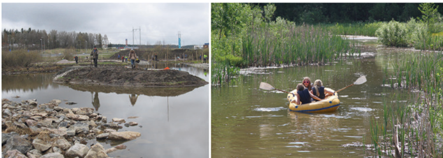
Fig. 10 The Nummela Gateway wetland park was constructed in 2010 by wintertime dry excavation, with some native trees planted on the site by an engaging volunteer event in May (left). In June 2013, the first children's summer camp was held at the site (right). Photograph Salminen (2010, 2013)
