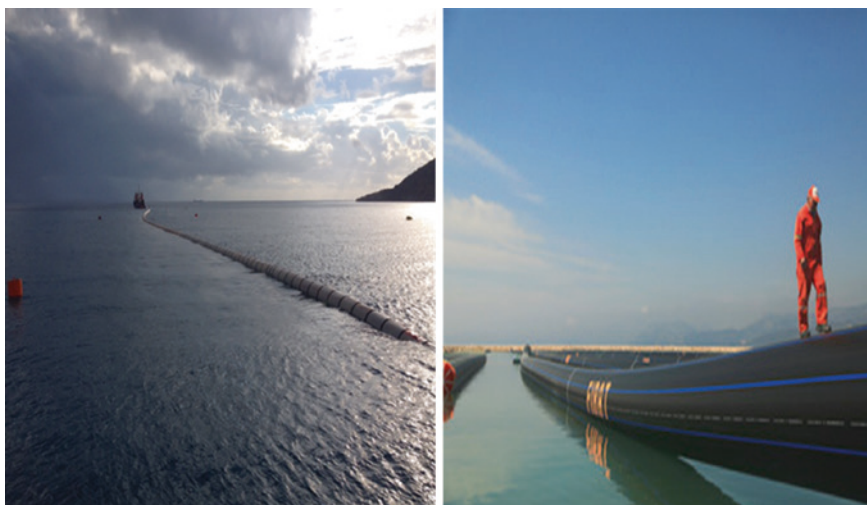
Fig. 13 The HDPE pipes used in the project
