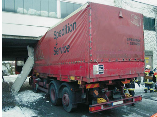
Fig. 2 Truck accident due to failure to observe the clearance height (Source: Karlsfeld fire service)
