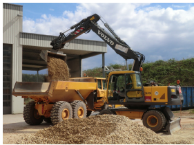
(a) Bucket excavator THOR
