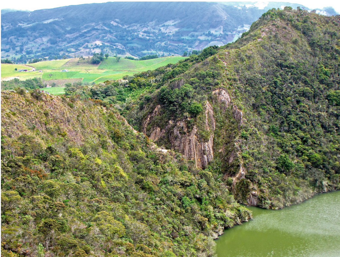
Fig. 9.3 Artificial drain cut in nineteenth century in the NW part of the lake. Gullying due to later surface erosion. Photography Michel Hermelin
