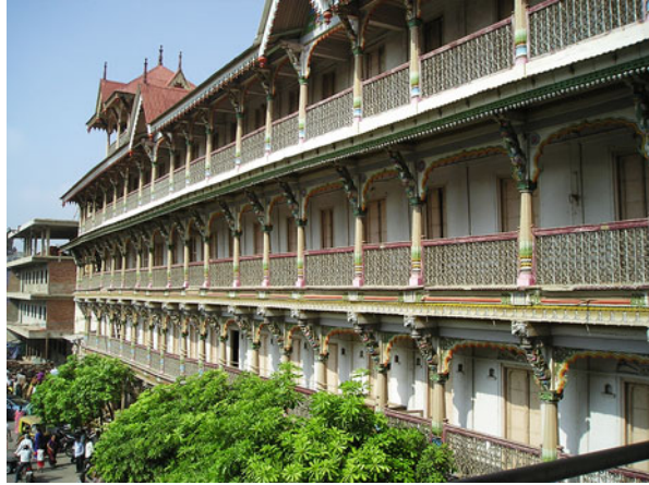
Fig. 10 Svāminārāyaṇa Temple (1822) Kalupur, Ahmadabad. Façade of the haveli for female devotees, constructed with ornate pillars and brackets with imagery of heavenly life and intricate carvings of the life of Kṛṣṇa ( Kṛṣṇa-līla ). Winged figures are found at different locations in the brackets. Photo by Rabindra J. Vasavada, June 2011
