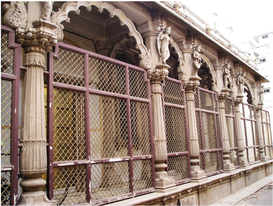
Fig. 1 Cintāmaṇi Parśvanāth Derasar (1798, renovated in 1904), Waghān Pōl, Ahmadabad. The temple's renovated façade is part of a long veranda space running along the street. The façade contains composite pillars with motifs that translate from Mughal architecture, and are suggestive of tapering trunks and crossed capitals supporting ornate, cusped arches which span the openings. The façade brackets support various angelic figures. Photo by Rabindra J. Vasavada, June 2011
