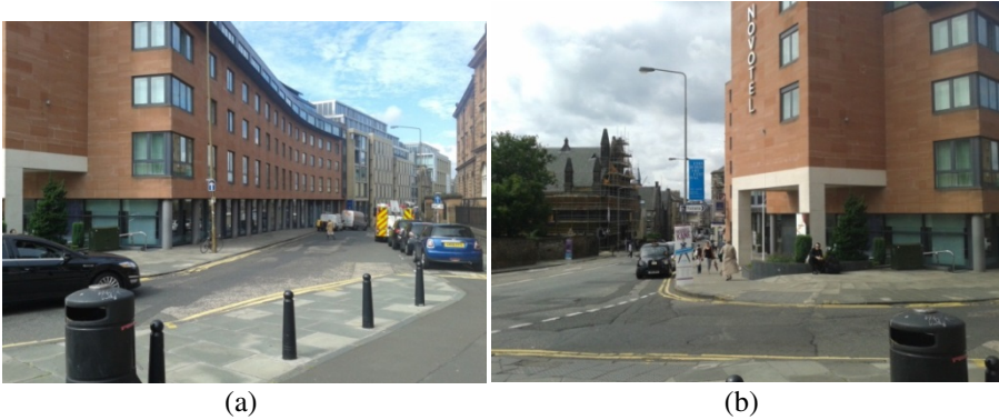
Fig. 6. The Novotel on Lady Lawson street and the absence of any street sign
