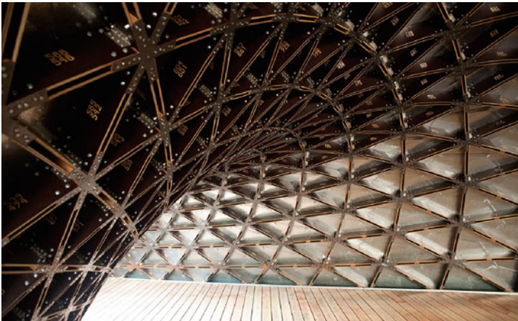
Fig. 8 A complex shape and pattern of a grid structure is achieved with no collisions between panels around nodes by taking advantage of panel thickness and spacer gaps between parallel panels
