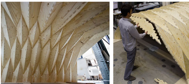
Fig. 1 Timber folded plate built from 21 mm LVL panels, assembled with single-degree-of-freedom dovetail joints without adhesive bonding. Components interlock with one another
