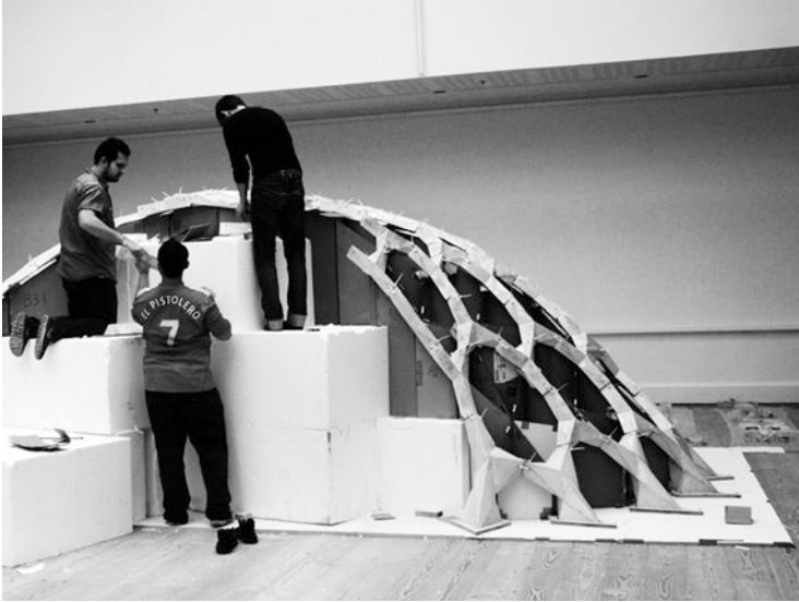
Fig. 3 In earlier experiments extensive falsework was needed for construction post-tensioning
