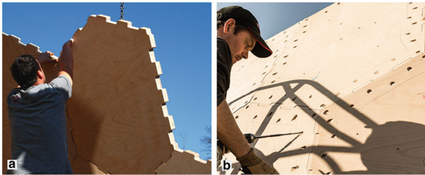
Fig. 10 (a) Assembly of a structural plywood plate. (b) The plates are fixed and held in place through the crossing screws
