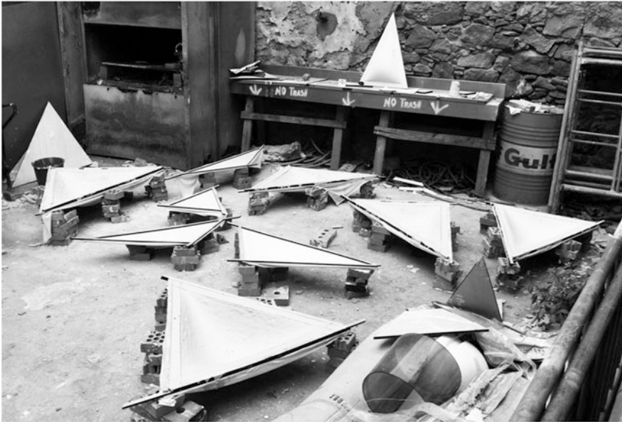
Fig. 5 Simple approach to uniquely cast tiles: plywood fabric formwork frames (Maxwell 2013)
