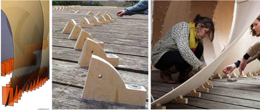
Fig. 11 Left : auxiliary sectioning planes (in vertical position) to determine the shapes of the wedges. Middle : photograph of the definite position of the wedges after setting out with the total station and the full-scale templates. Right : installation of nylon cable ties to link the wooden surfaces to the wedges
