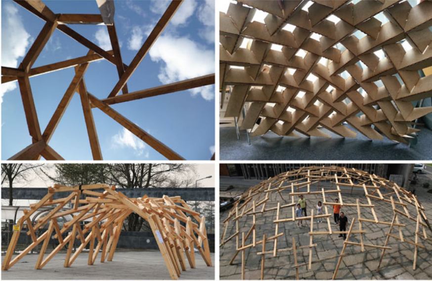
Fig. 1 Physical RF-structures designed and fabricated by architects: a simple roof structure ( top-left ), a design by Michael Clarke ( top-right ), a design from Spiro-ETH ( bottom-left ), and a design from Wan Shu and Kengo Kuma ( bottom-right )
