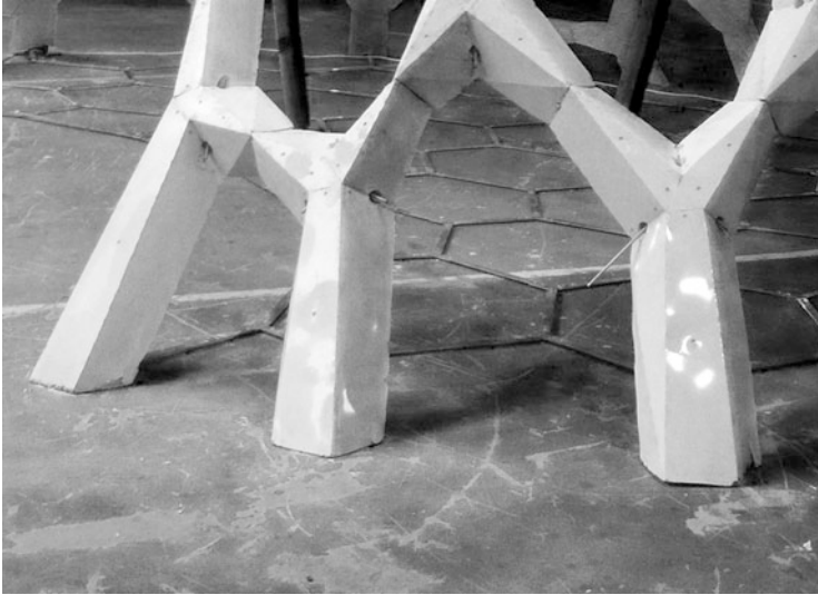
Fig. 11 Geometry change in base elements
