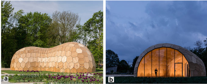
Fig. 12 Photographs of the finished prototype building
