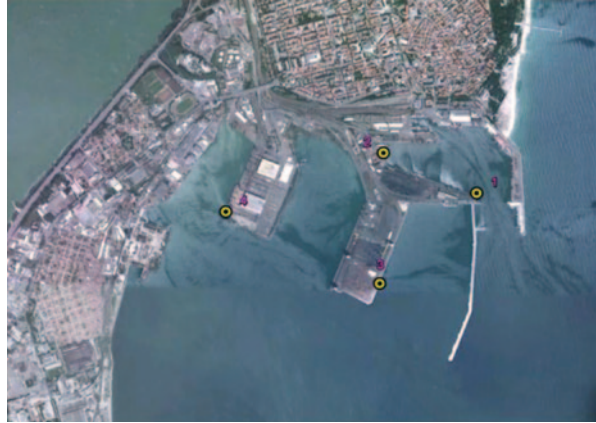
Fig. 3.1 The port of Bourgas. PM10 monitoring is performed at site 2. The hypothetical open area source used for AERMOD dispersion calculations is north of site 3
