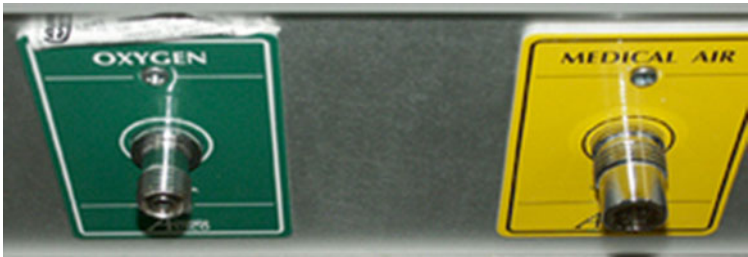
Figure 10.2 Diameter index safety system
