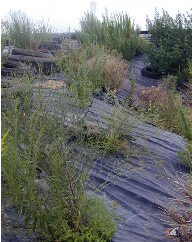
Fig. 5.2 Spontaneous plants growing on an unclosed landfill in Buenos Aires province temporarily covered with a plastic liner
