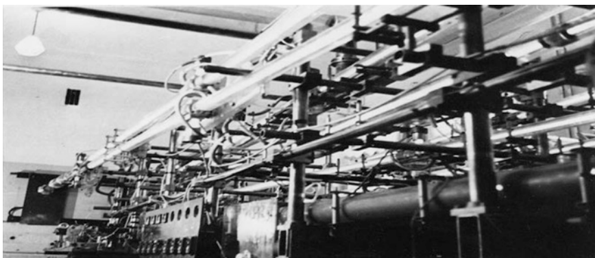
Fig. 15.2 “Zig-Zag”— \text{CO}_2 -laser created by A.I. Barchukov FIAN 1970 [2]
