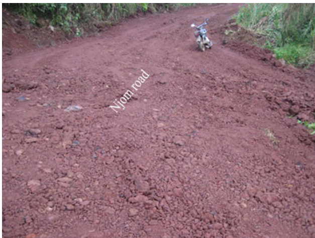
Fig. 21 Coating of road with the pouzzolana in the Njom Village
