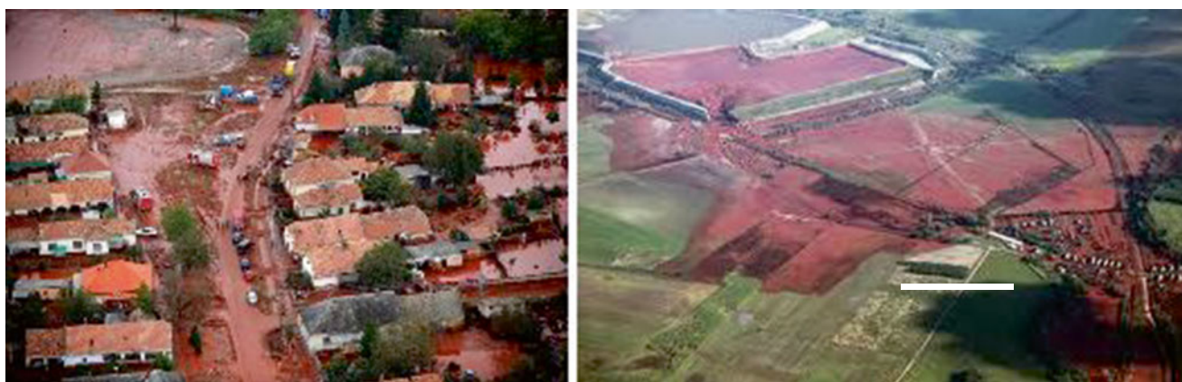
Fig. 1.6 Aerial photographs of the Ajka alumina waste pond, Veszprém County, Hungary (photographs 1 and 2) (source of photograph 1: http://mysterytricycle.com/wp-content/uploads/2010/10/Sludge.jpg ) (source
