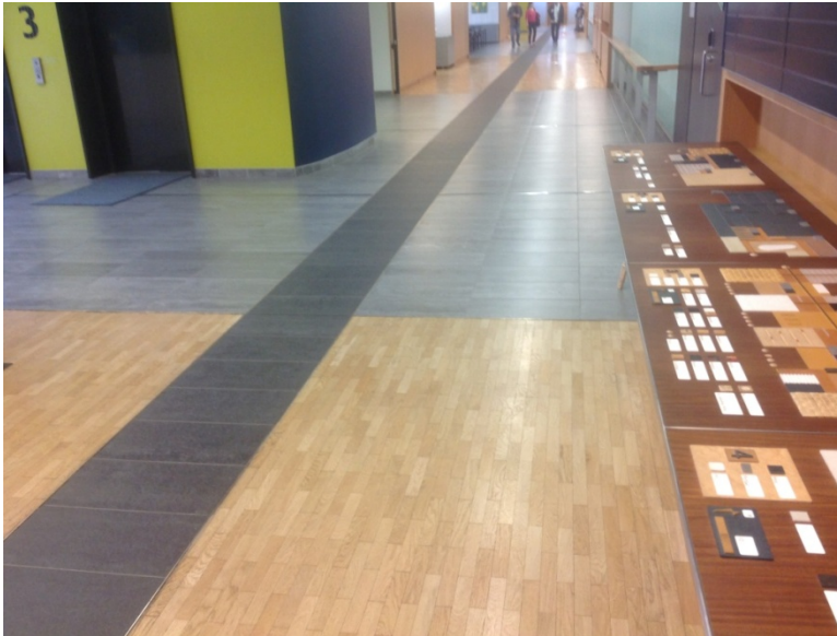
Fig. 3. General lobby area with safety related features. Please note changes in contrasts, different materials and tactile route markers that guide to the exits.
