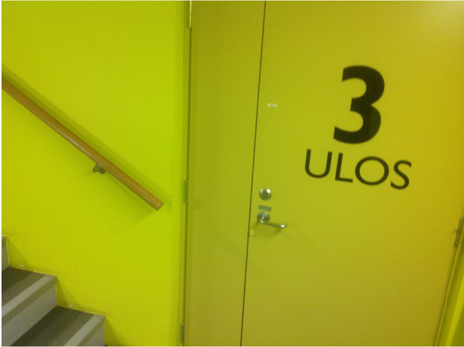
Fig. 1. Exit door. Please note large size number 3 as well as number three written in Braille on top of the door handle near to the handle itself. On the hand-rail there are three wooden buttons to denote third floor.
