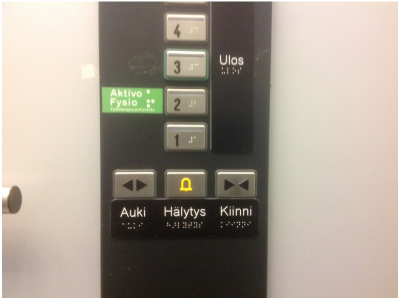
Fig. 2. Safety features in an elevator. Please note the bell button and raised symbol as well as raised exit floor buttons.
